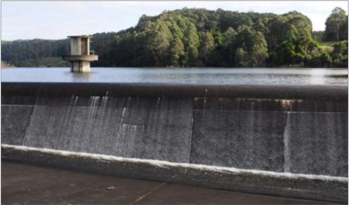
Figure 3. West Barwon Reservoir spillway.
