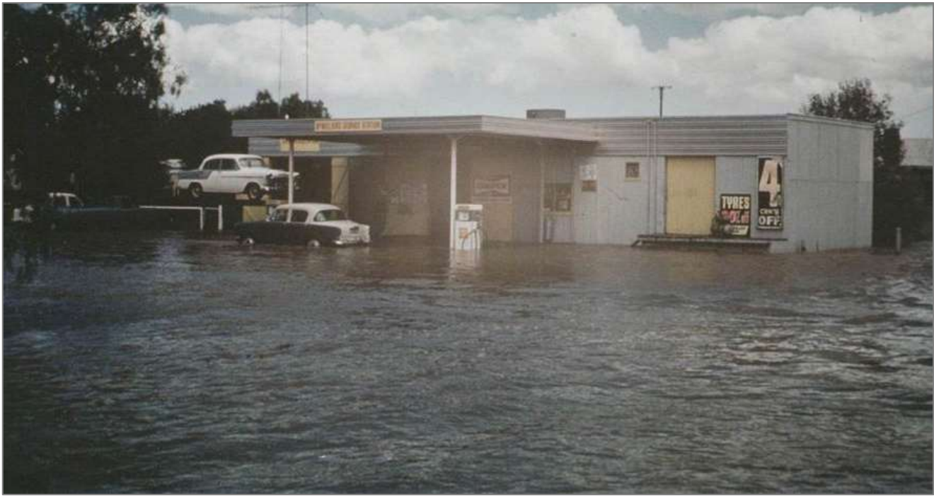
Figure 9. Flooding impacting the Inverleigh Service Station, 19 High Street during the 1973 flood event.
