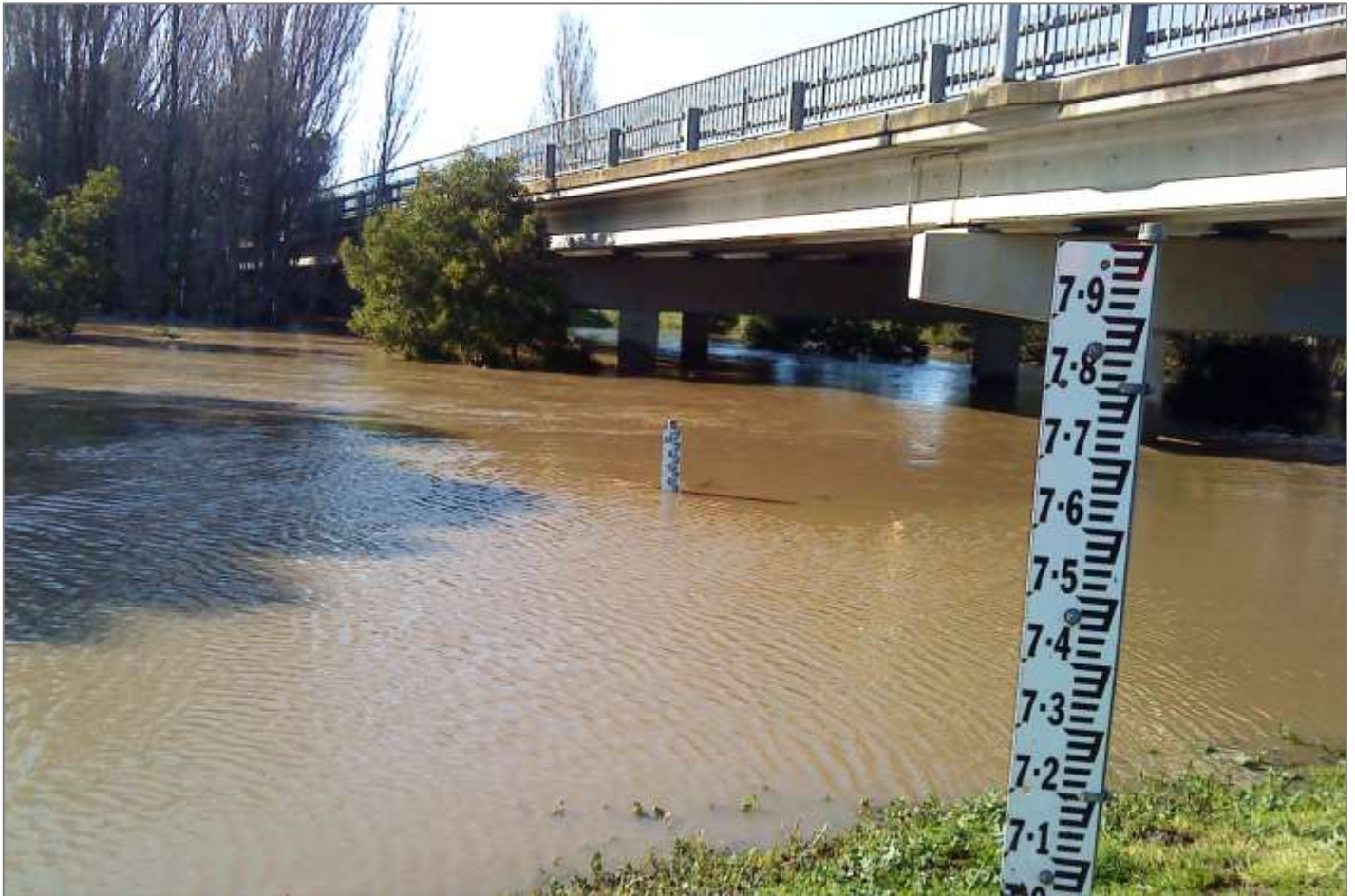
Figure 35. Shelford gauge boards adjacent to the Bannockburn-Shelford Road bridge during the 2011 flood event (source: Nathan Hansford)
