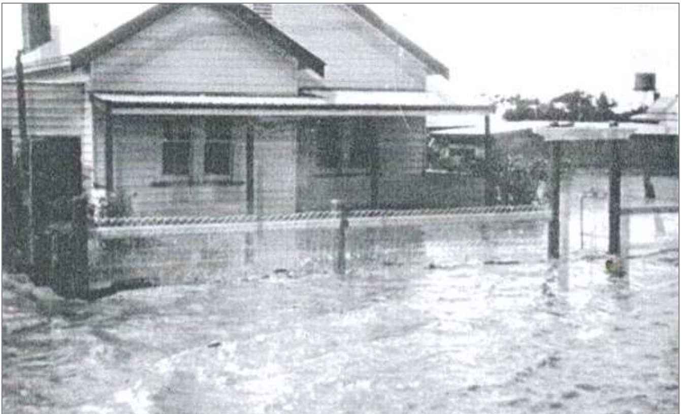
Figure 8. Flooding surrounding a house in Dundas Street, Inverleigh during the 1973 flood event.
