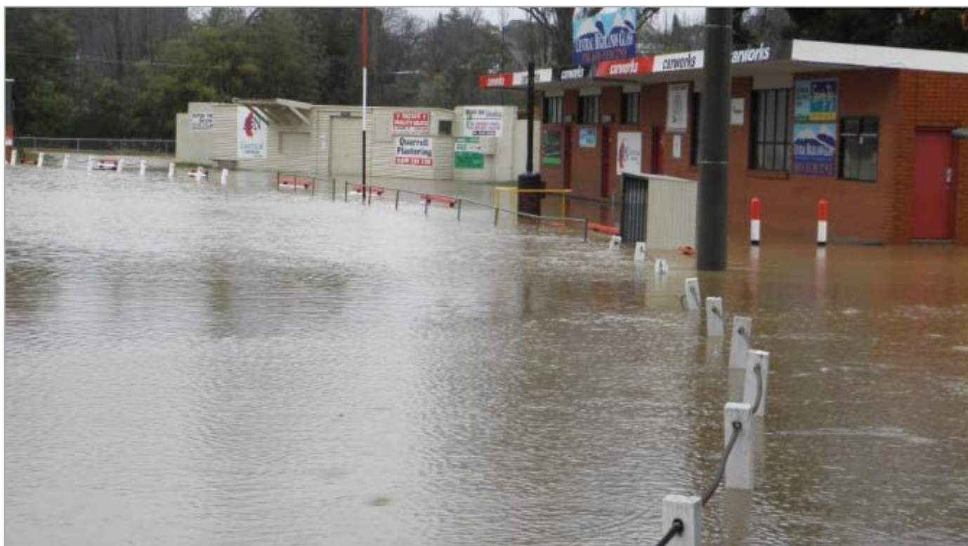
Hammon Park impacted by flooding during the January 2011 flood event.
