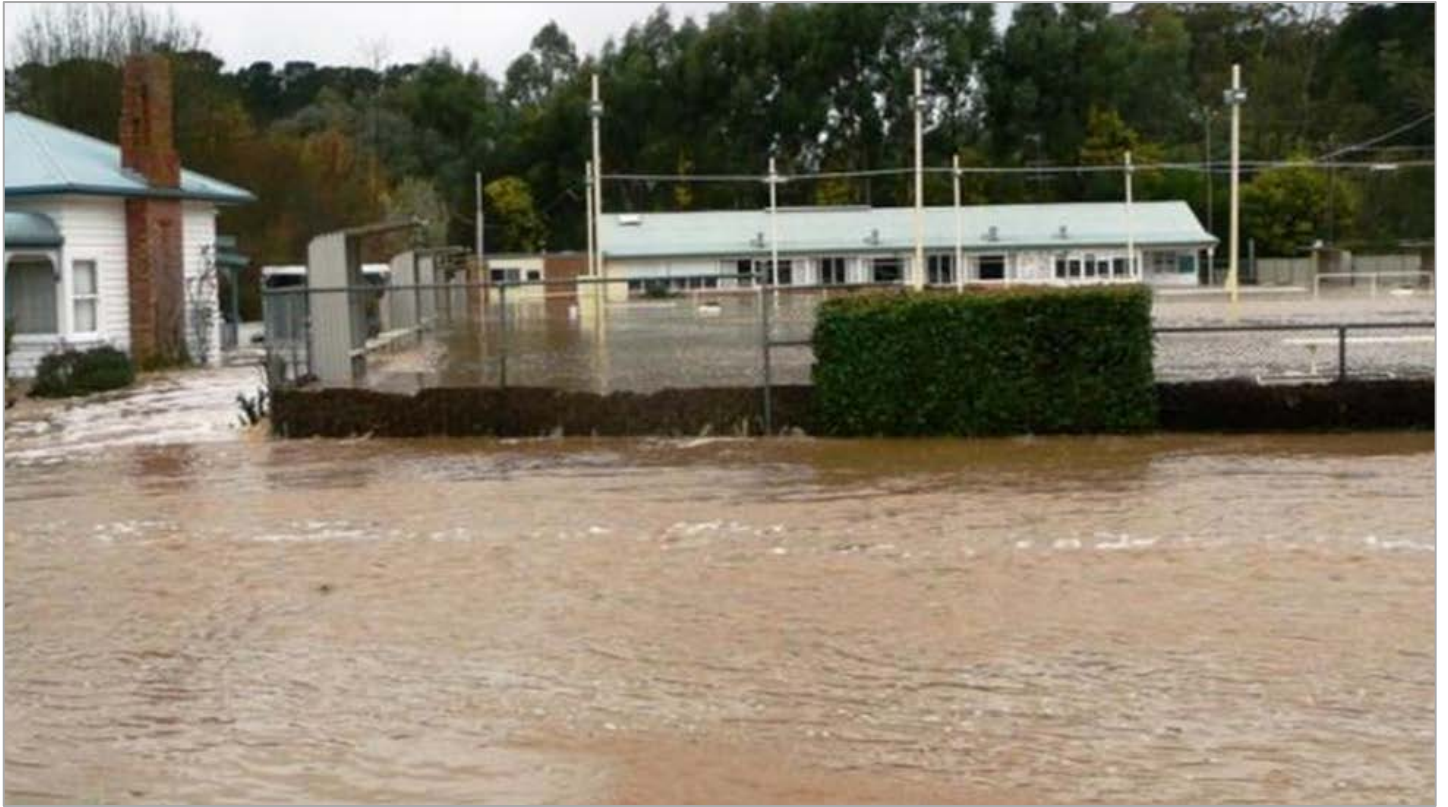
Creswick Bowling Club impacted by flooding during the January 2011 event.
