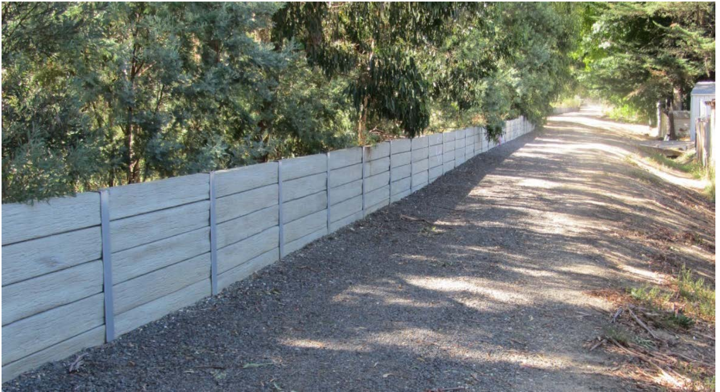
Creswick levee wall, looking upstream from Castlemaine Road.
