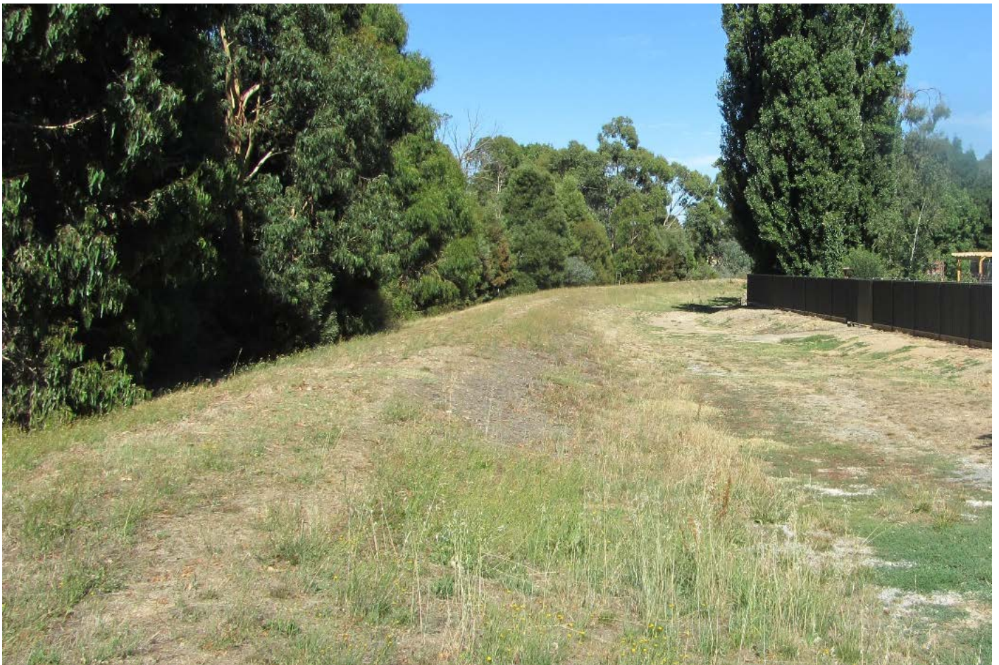
Creswick levee at the rear of properties along Castlemaine Road.
