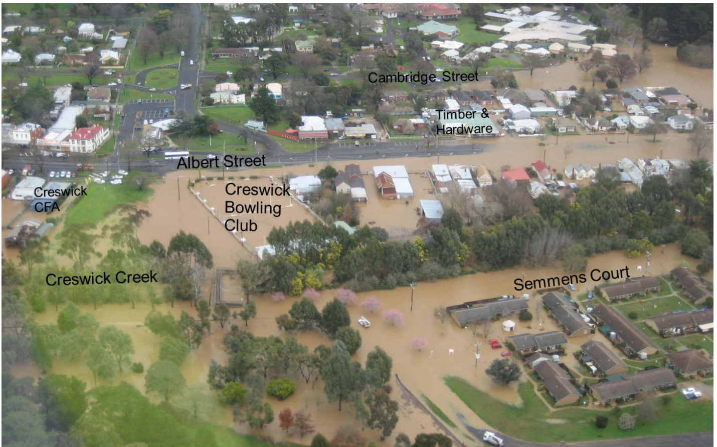
Creswick looking west along Albert Street during the September 2010 flood event (NC CMA).
