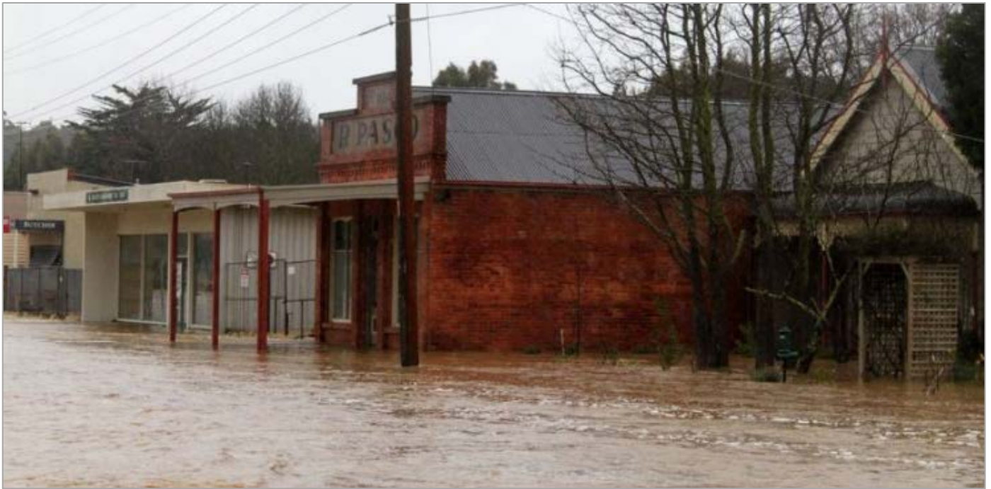
Buildings impacted by flooding along Albert Street in Creswick during the January 2011 event.
