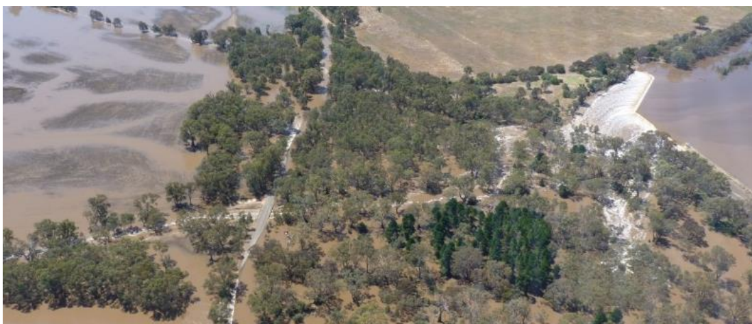
Lake Lonsdale spilling during January 2011 flood event.
