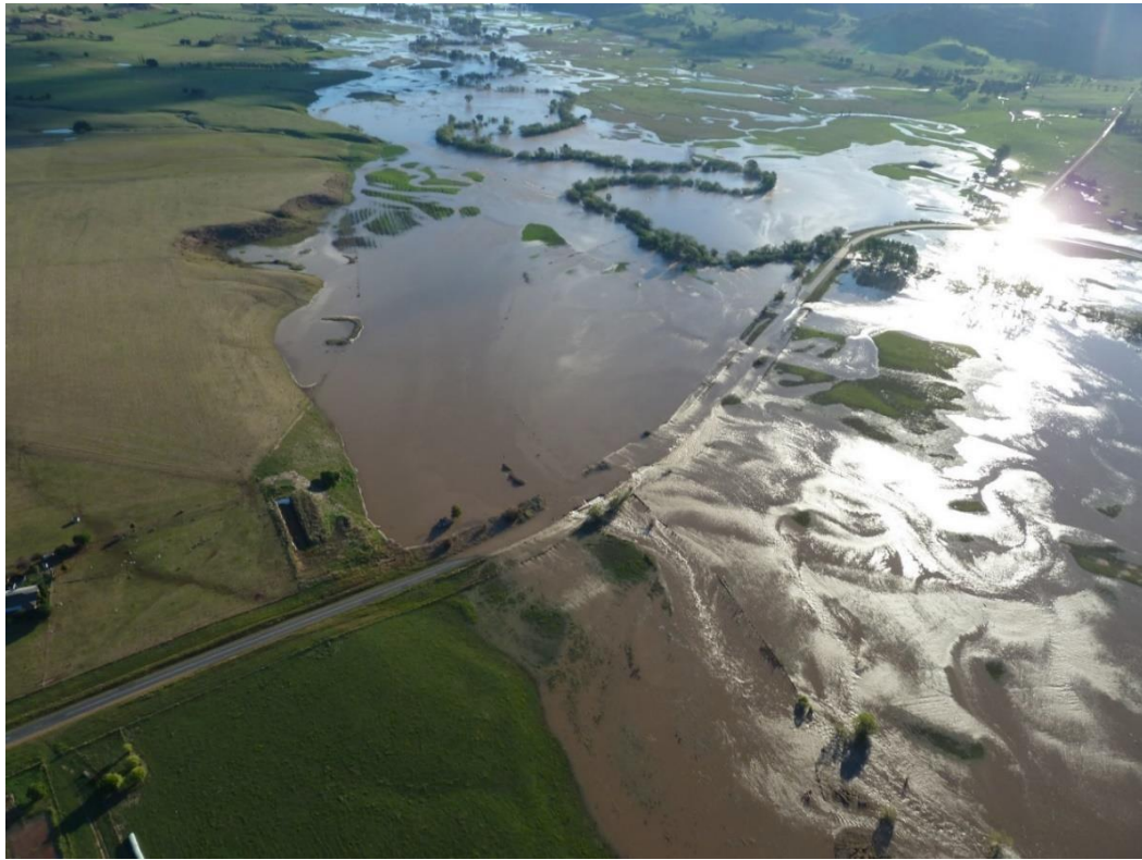
Figure 12 Murray River Road at Tintaldra - looking upstream on Cudgewa Creek (March 2012, after flood peak)
