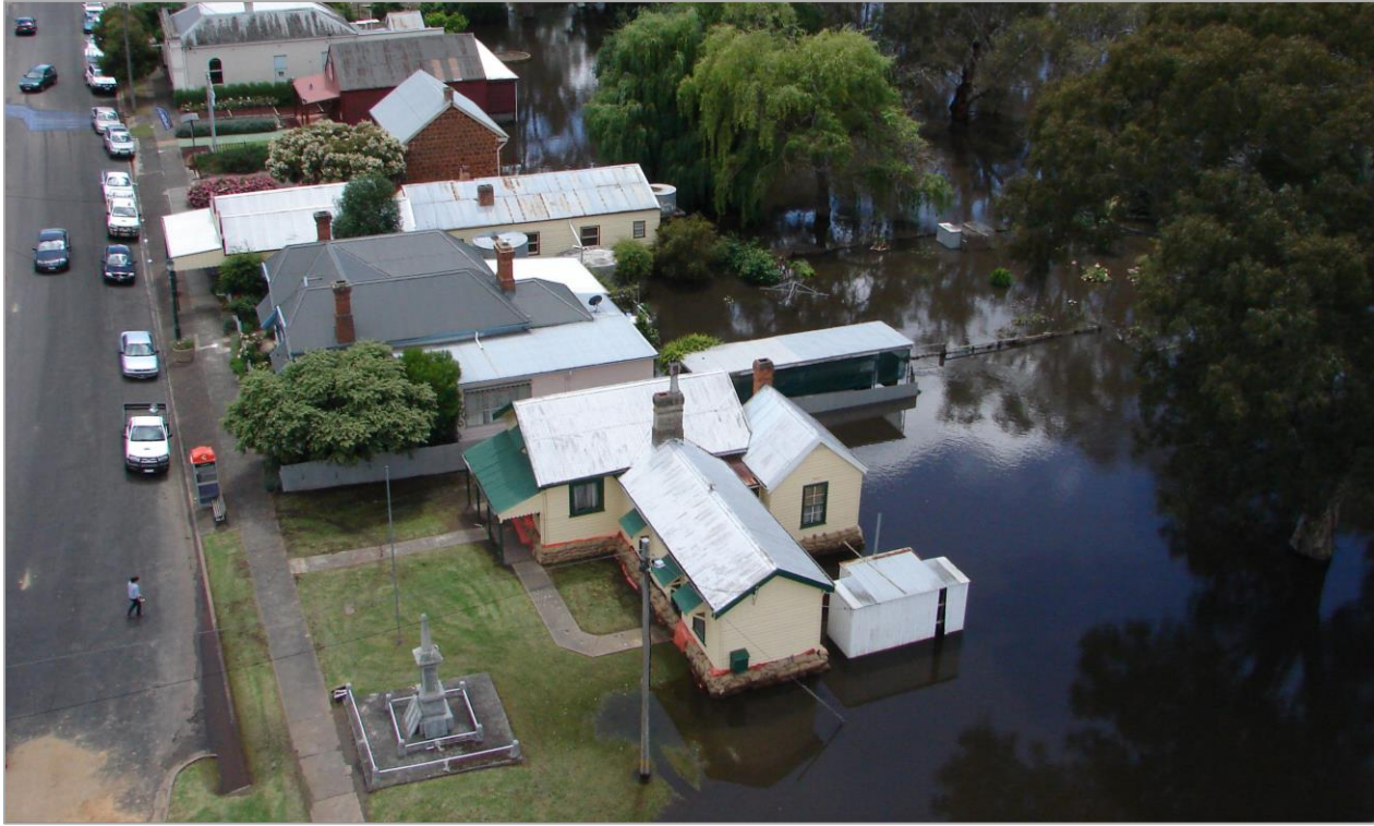
RSL building in Bair Street, Harrow in December 2010
