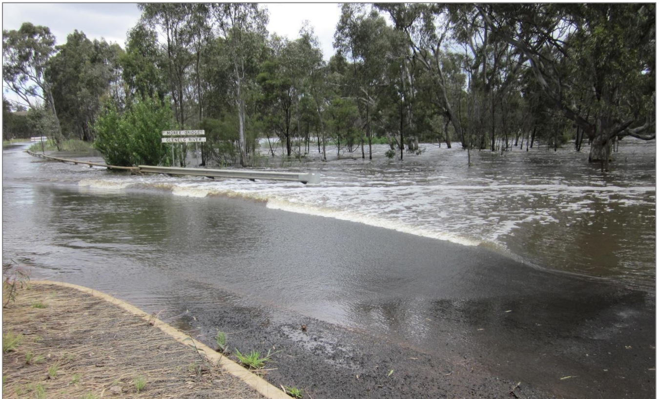
Flooding overtopping the Moree Bridge, downstream of Harrow in December 2010
