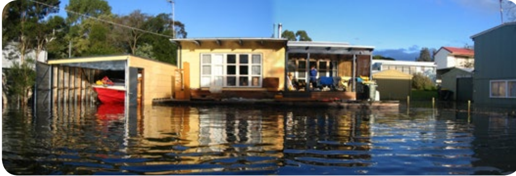
Flooding in Gippsland Lakes, June 2007
