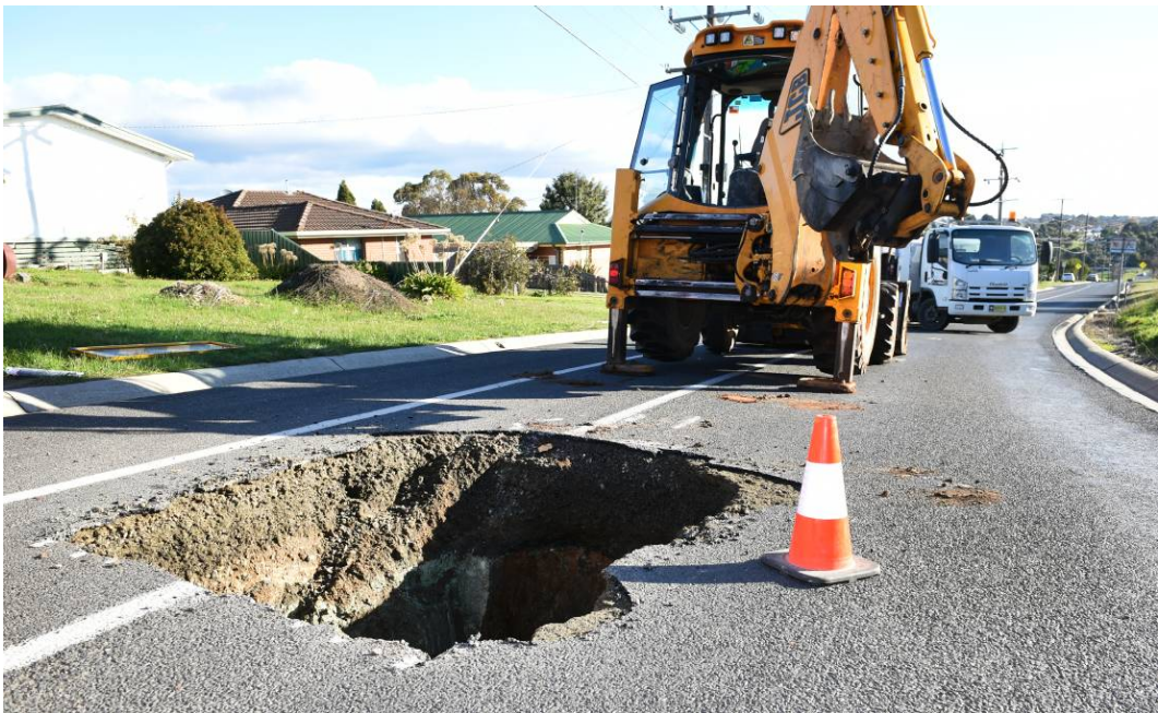
Photo 8. June 2018, a mine ventilation shaft collapsed in Elsworth Street, Mt Pleasant (source: The Courier).
