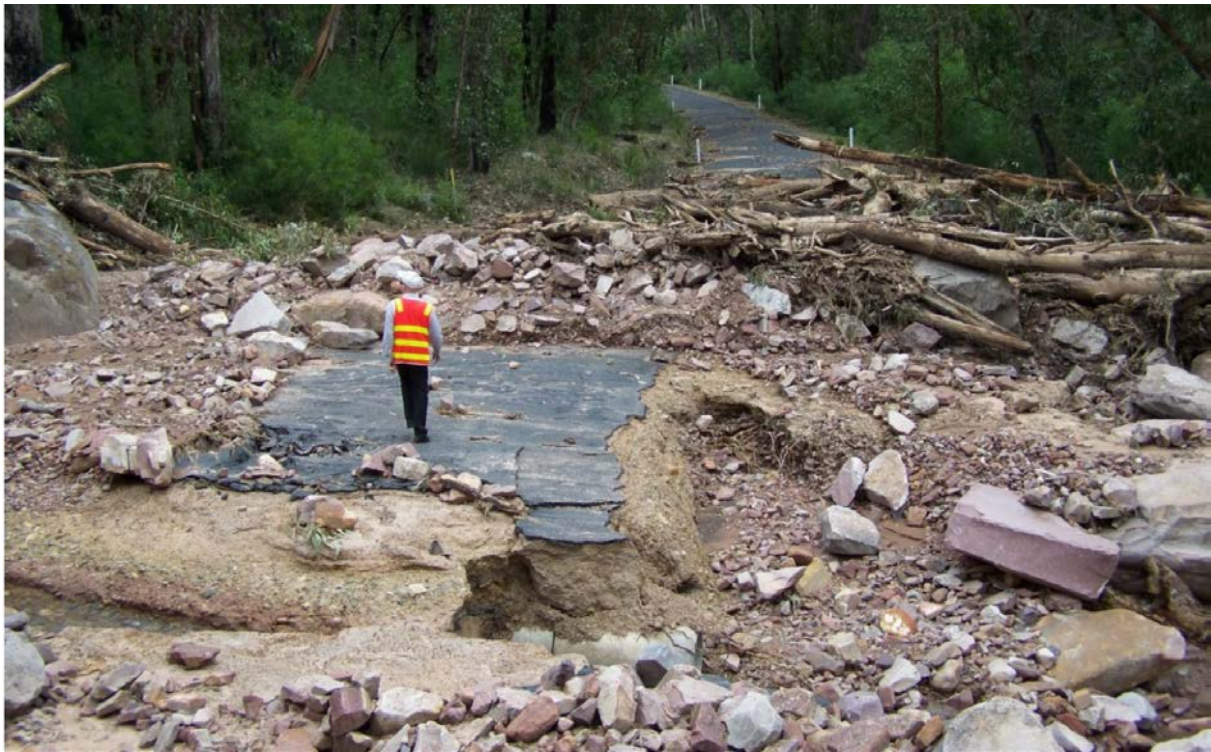
Photo 3. Damage to Silverband Road and culvert damage caused by January 2011 landslides (source: Vic Roads).
