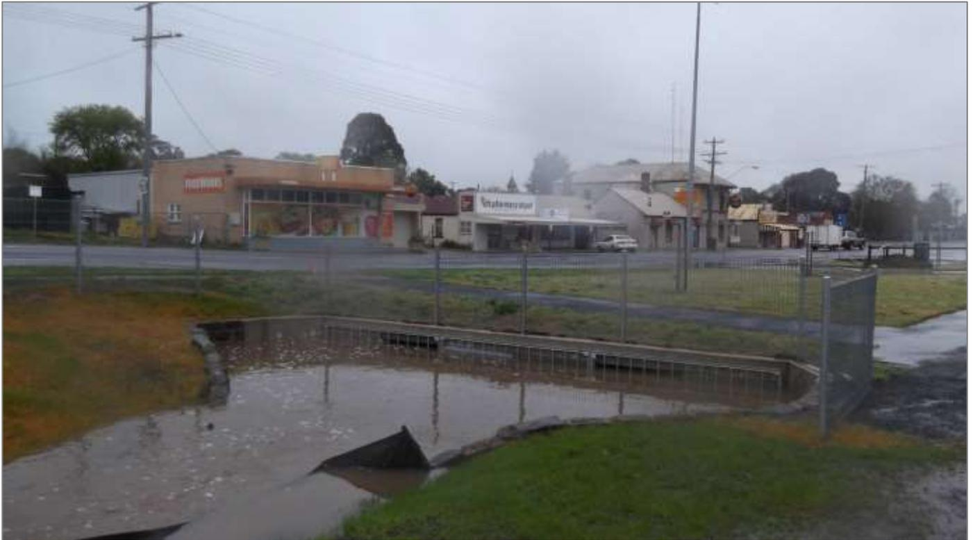
Figure 4. New culverts in Montgomery Street, during the September 2016 flood event.
