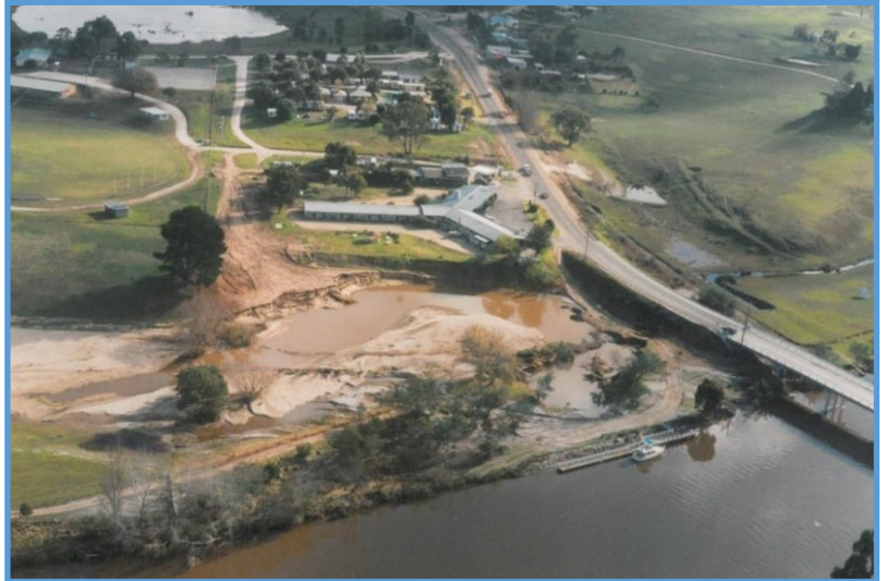
Image: Swan Reach Hotel, bank erosion. 1998. DELWP .
