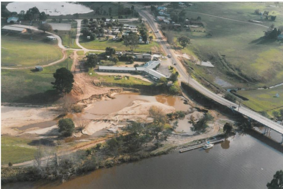
Bank erosion and remaining pools at the Swan Reach Hotel, indicating the height and extent of the floodwaters (DELWP, 1998)
