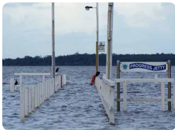
Paynesville Jetty, 2007 flood
