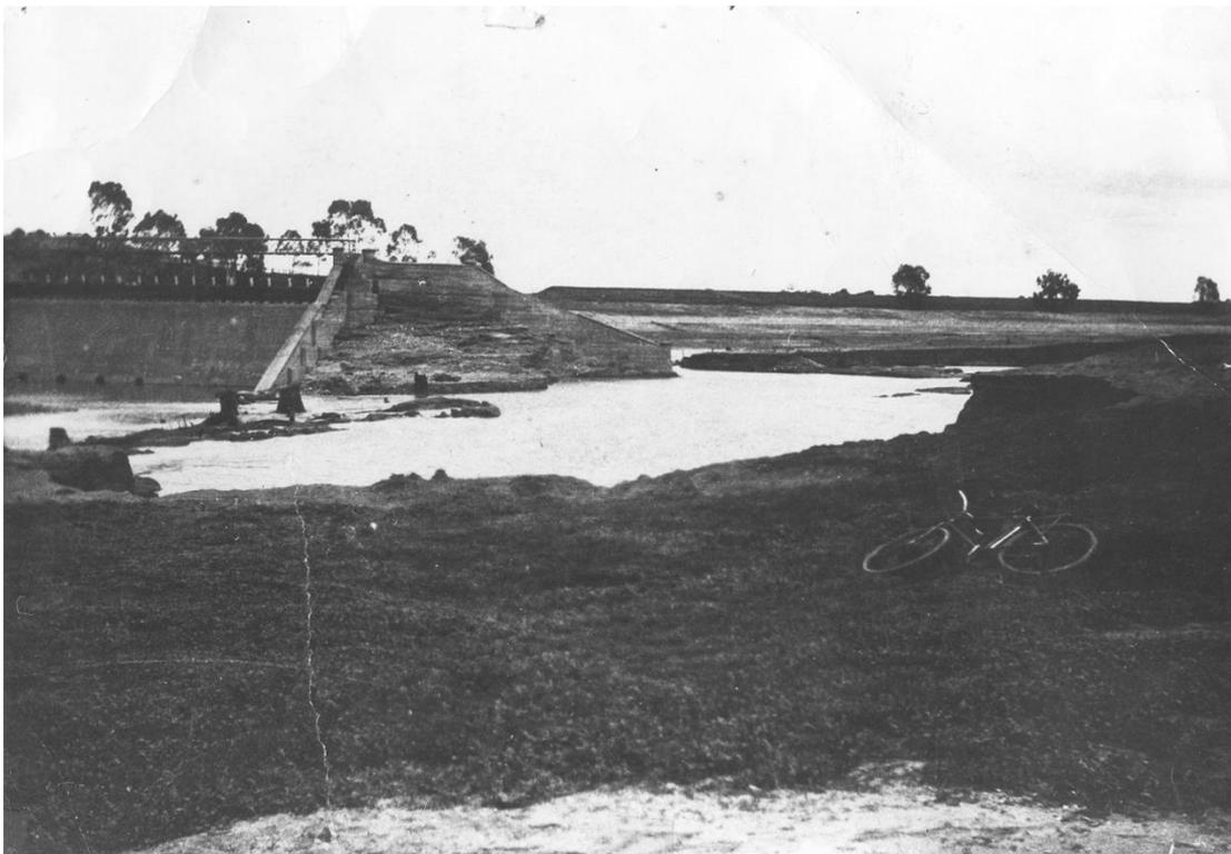
*Picture above: Laanecoorie Reservoir Dam Wall Failure, 1909*
