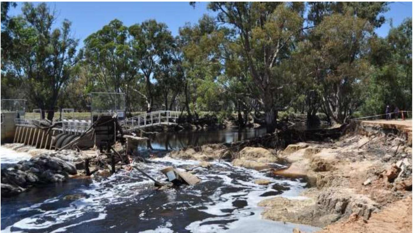
Figure 22. The Dimboola Weir damaged by flooding during the 2011 flood event.
