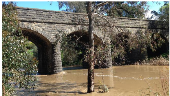
Deep Creek at Bulla Bridge
