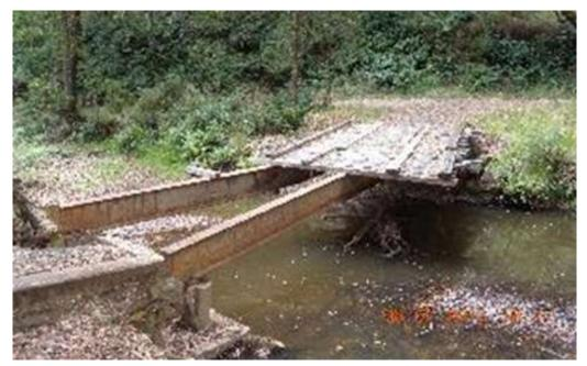
Figure 74. Damage to the Martin Street Bridge in Blackwood following the 2010 flood event.
