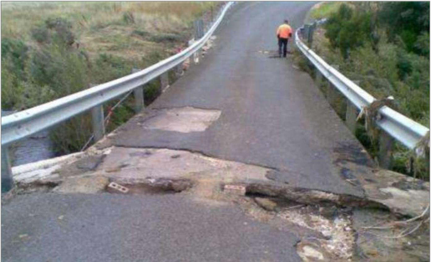
Figure 51. Flood damage to Dehnerts Road (north-west of Ballan) caused by the January 2011 flood event (Melbourne Water 2013).
