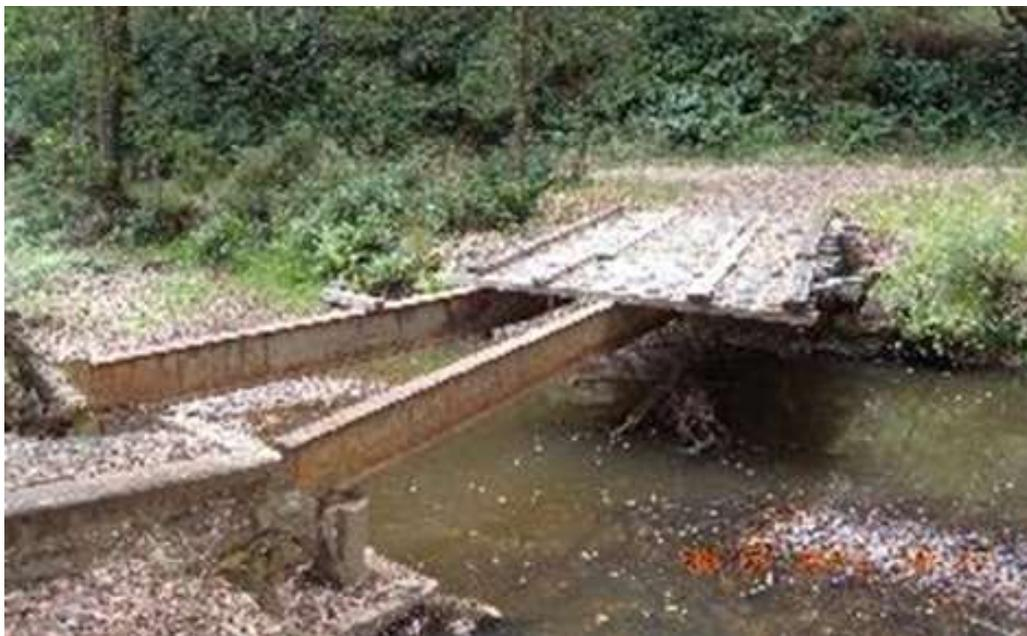
Figure 74. Damage to the Martin Street Bridge in Blackwood following the 2010 flood event.
