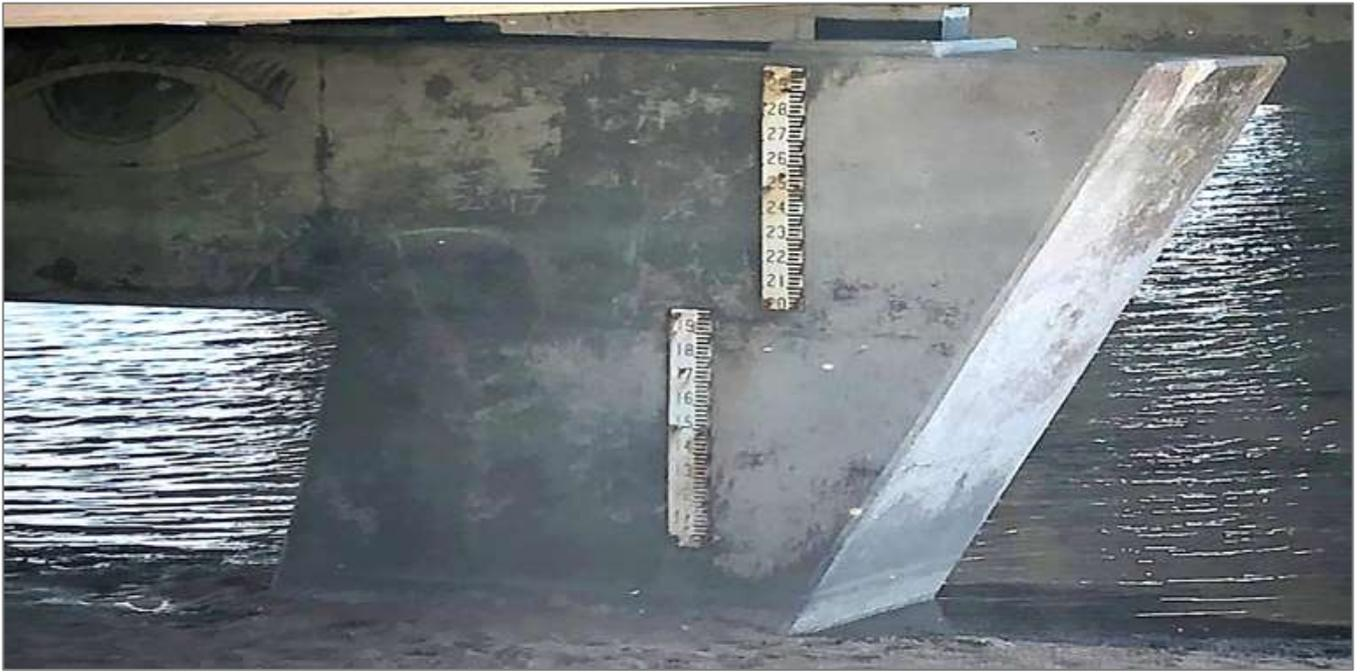
Figure 37. Curdies Inlet gauge board on the Peterborough Bridge.
