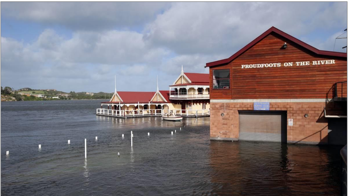
Figure 63. Flooding from the Hopkins River impacting the Warrnambool Rowing Club in Simpson Street during the 2014 flood event.
