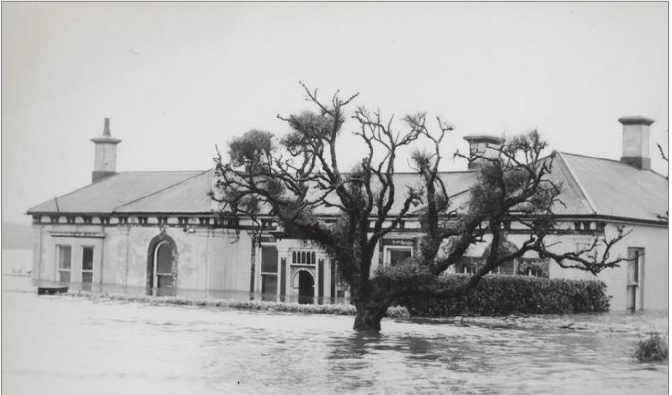
Figure 25. Flooding impacting a house near the Botanical Gardens, Cox's House during the 1946 flood event.
