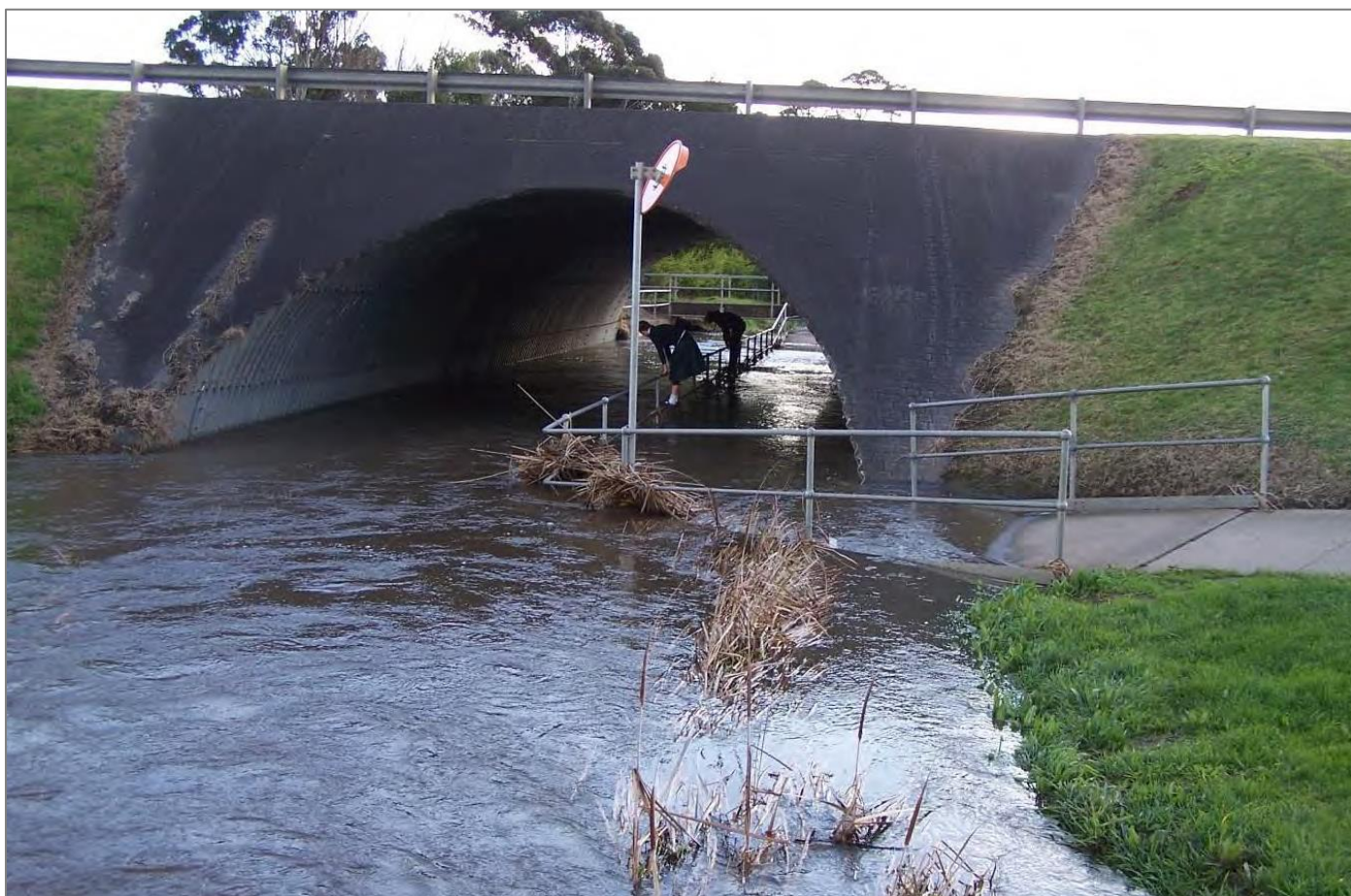
Figure 15. Mortlake Road culvert before the culvert upgrade, 12 th August 2010 (Utilis, 2018).
