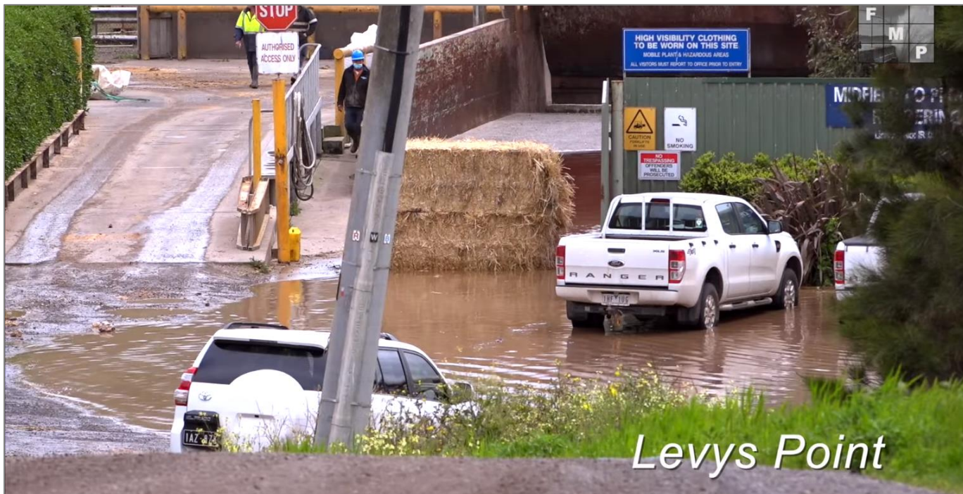
Figure 28. Flooding impacting the Midfield Meat Rendering Plant during the October 2020 event.
