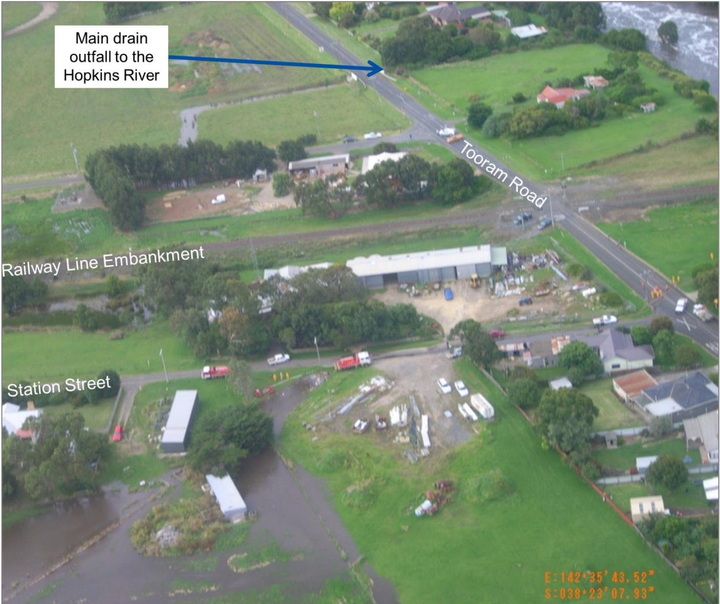
Figure 52. Buildings impacted by flooding in Allansford during the January 2011 flood event.
