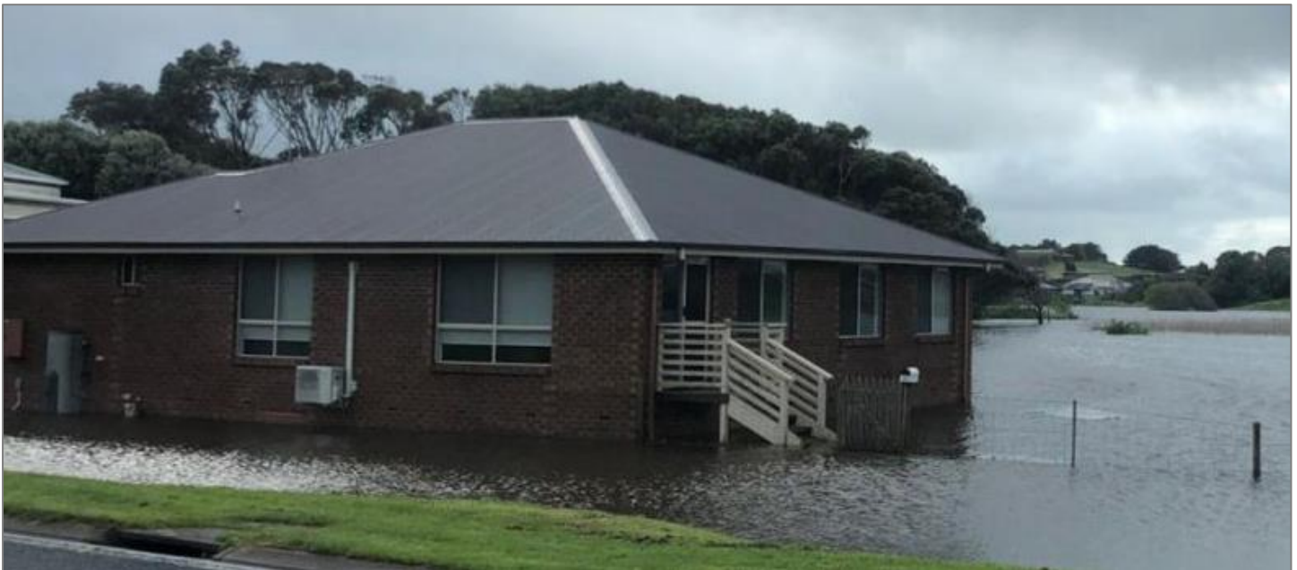
Flooding impacted a house at 6 Morse Road during the October 2020 event.
