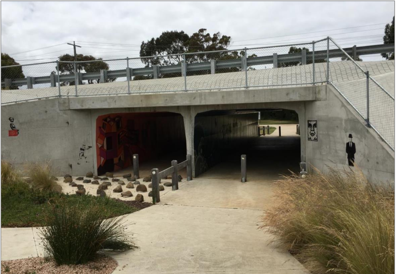
Figure 16. Mortlake Road upgraded culvert capacity to reduce flood risk (Water Technology, 2017).
