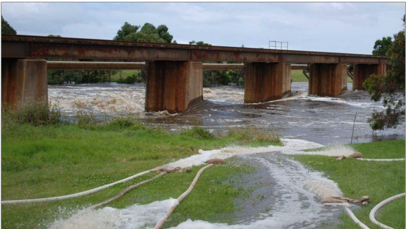
Figure 59. Pumping stormwater back into the Hopkins River during the October 2020 flood event.
