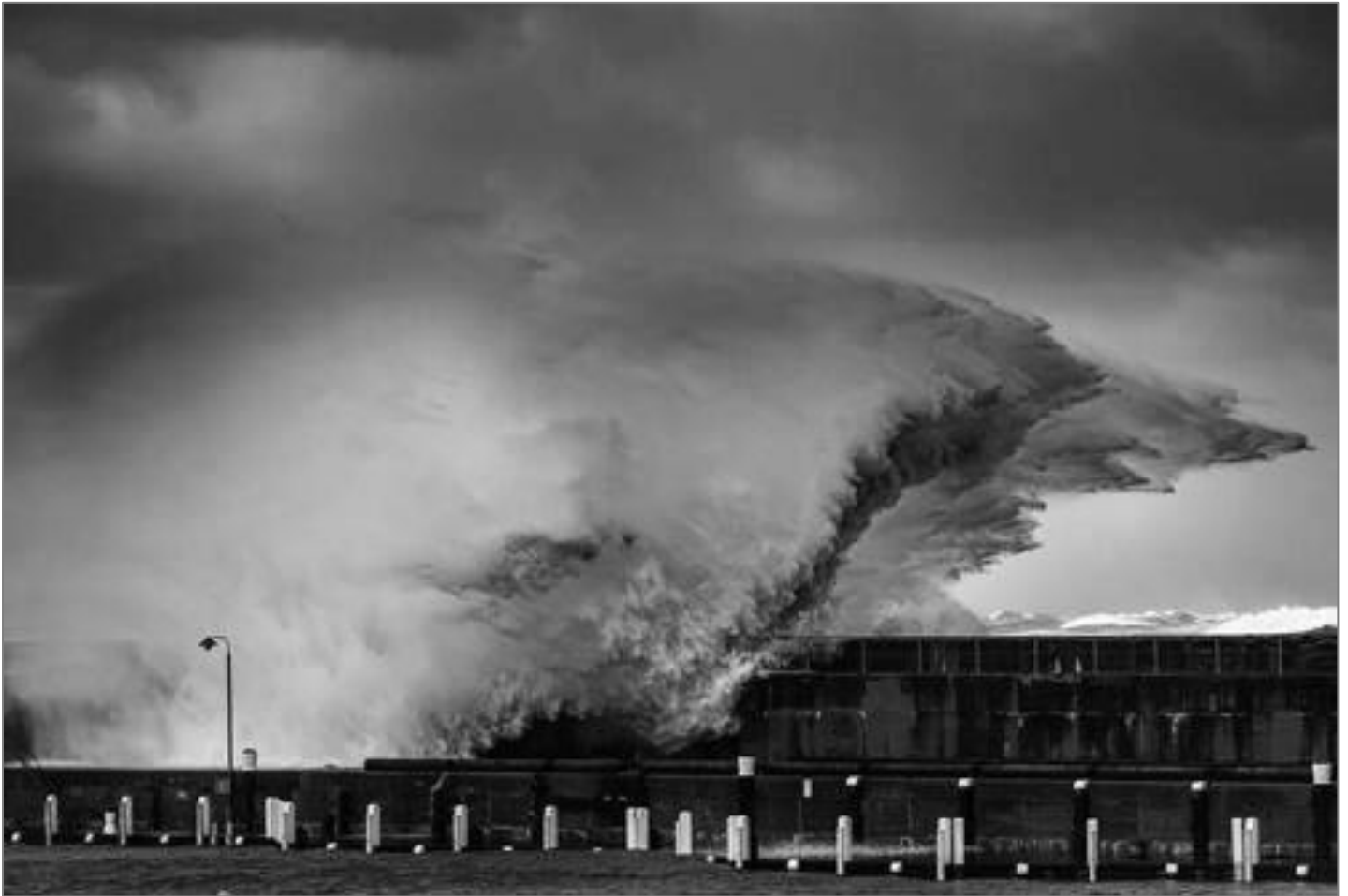
Figure 37. Storm surge event impacting the Breakwater Pier during the October 2014 event (ABC website).
