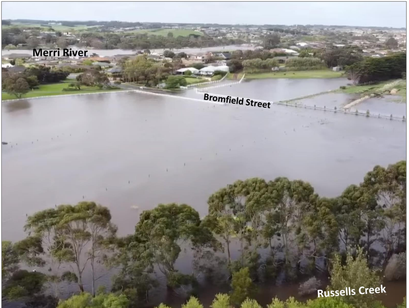
Figure 36. Flooding impacting the Bromfield Street, Warrnambool during the October 2020 flood event.
