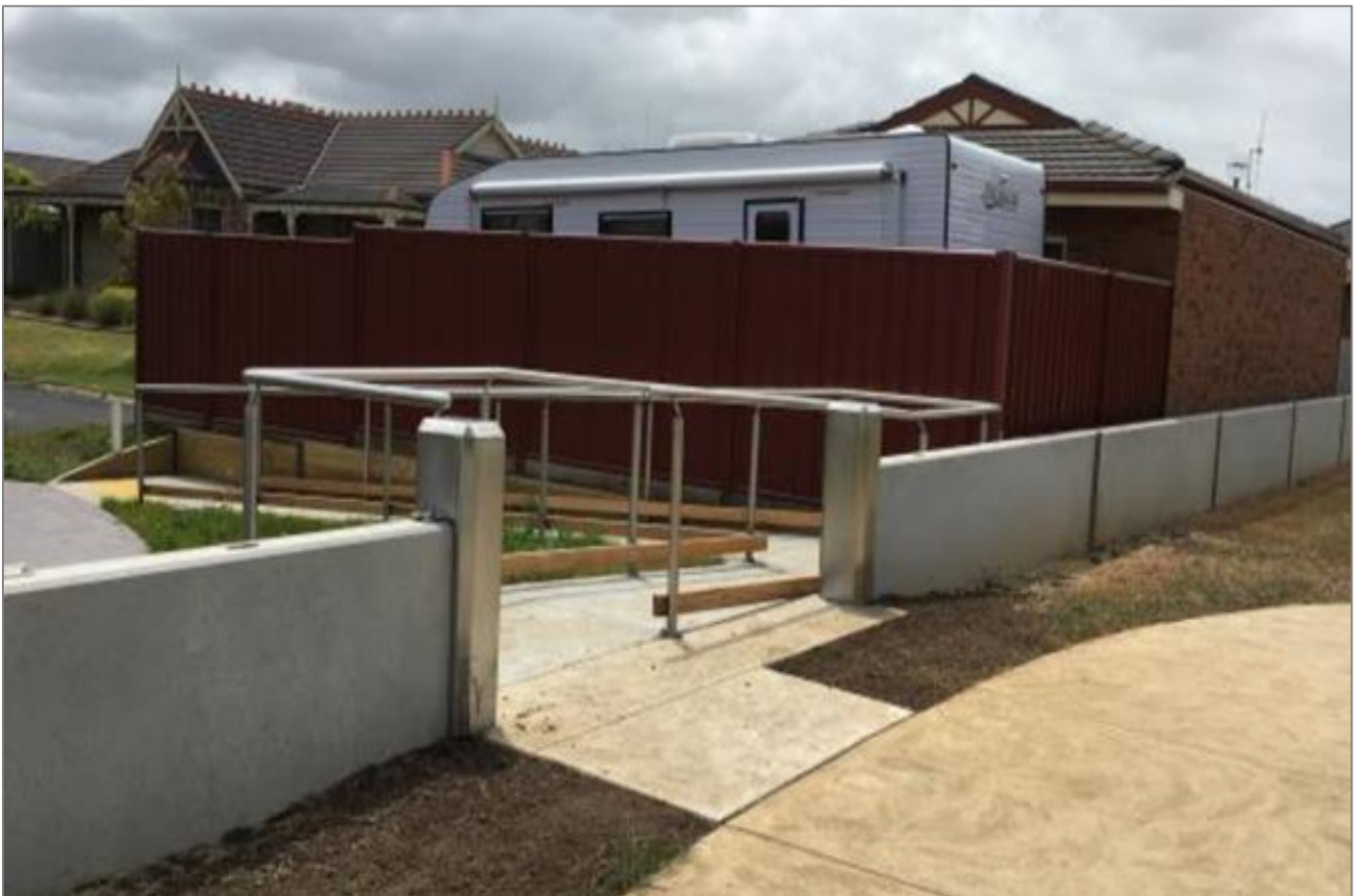
Figure 17. Russells Creek levee adjacent to Roslyn Close.
