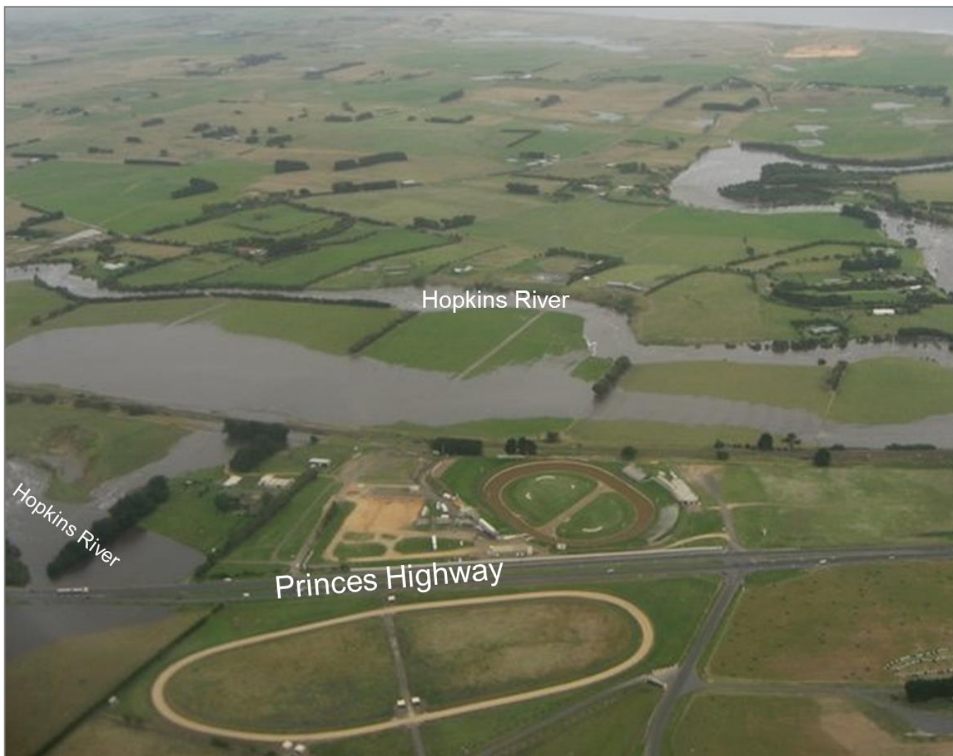
Figure 50. Flooding starting to impact the Princes Highway, west of Allansford during the January 2011 flood event.
