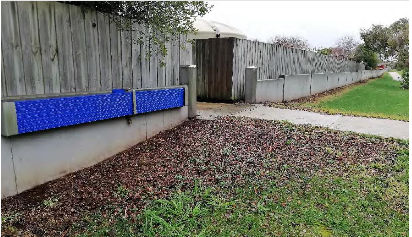
Figure 18. Russells Creek levee drop boards attached to the levee wall.
