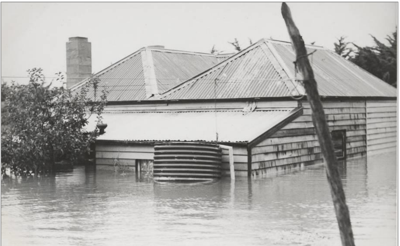
Figure 26. Flooding impacting a house in Broomfield Street during the 1946 flood event.
