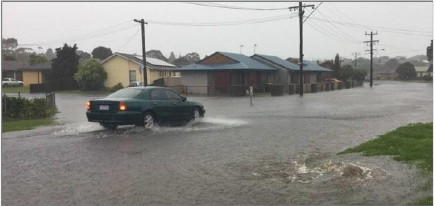
Figure 9. Flooding impacting properties along Wanstead Street during the October 2017 event (Utilis 2018).
