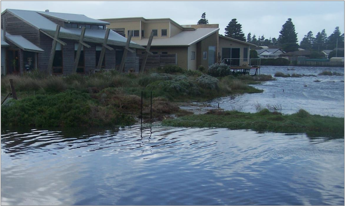
Figure 41. Buildings along MacDonald Street impacted by storm tide flooding during the June 2014 event.
