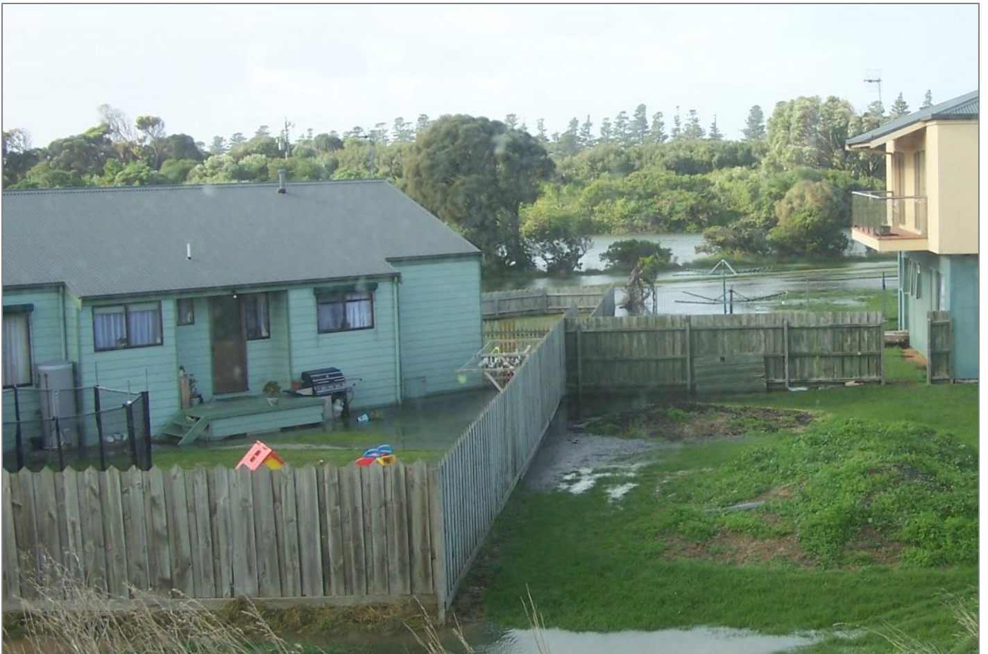
Figure 42. Buildings adjacent to the Merri River impacted by storm tide flooding during the June 2014 event.
