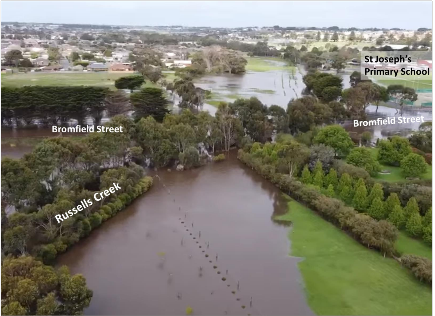
Figure 32. Flooding impacting the St Joseph's Primary School in Bromfield Street, Warrnambool during the October 2020 flood event (VICSES Warrnambool Unit).
