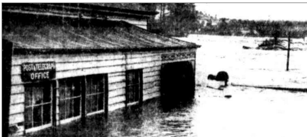
Figure 24. Woodford Post Office impacted by flooding during the 1946 flood event.
