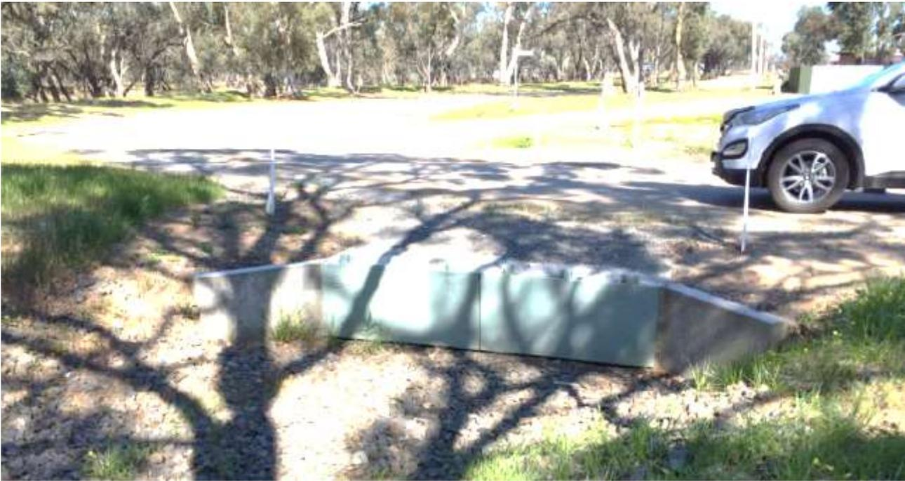
One way culvert flap valves at Asquith Reserve/McIntyre Street Warracknabeal Weir Pool eastern culverts
