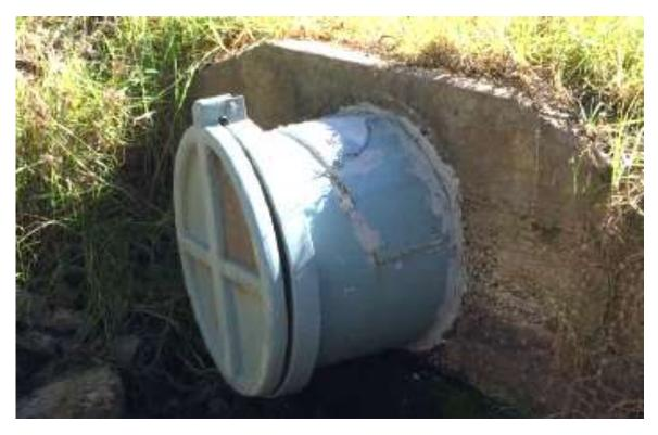
One way flap valve on a stromwater drain at Lyle Street Warracknabeal Weir Pool eastern culverts (Water Technology 2016).
