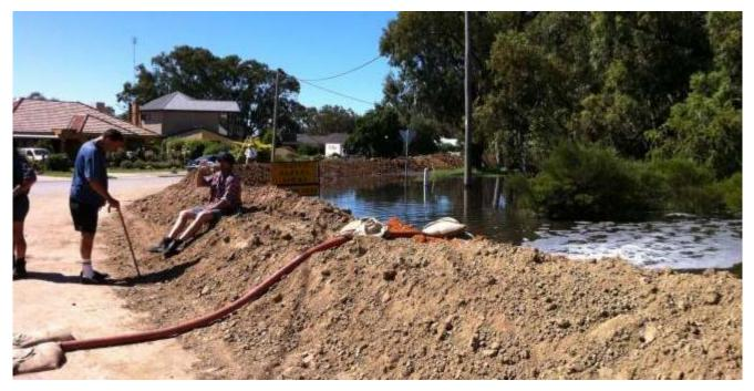
The temporary earthen Warracknabeal Levee constructed during the January 2011 flood event.
