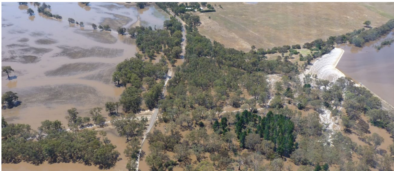
Figure 11. Lake Lonsdale spilling during the January 2011 flood event.
