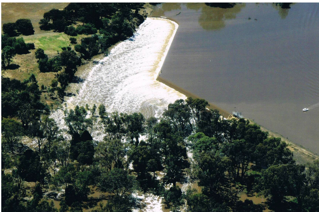
Figure 12. Lake Lonsdale spilling during the January 2011 flood event.
