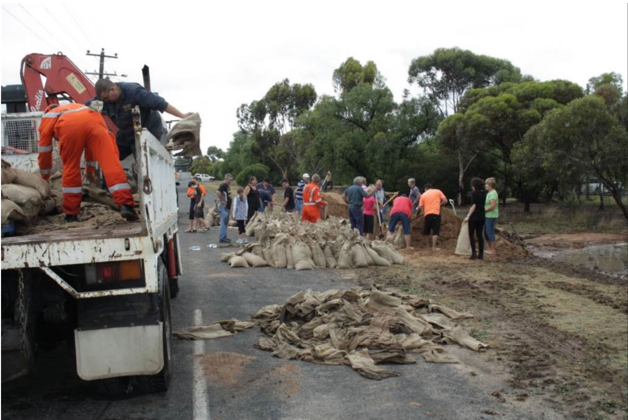
Figure 16. Sandbagging Natimuk Jan 2011
