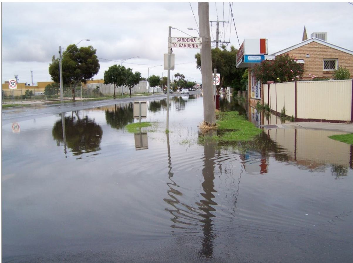
Figure 20. Flooding Gardenia St, Horsham during the January 2011 event.
